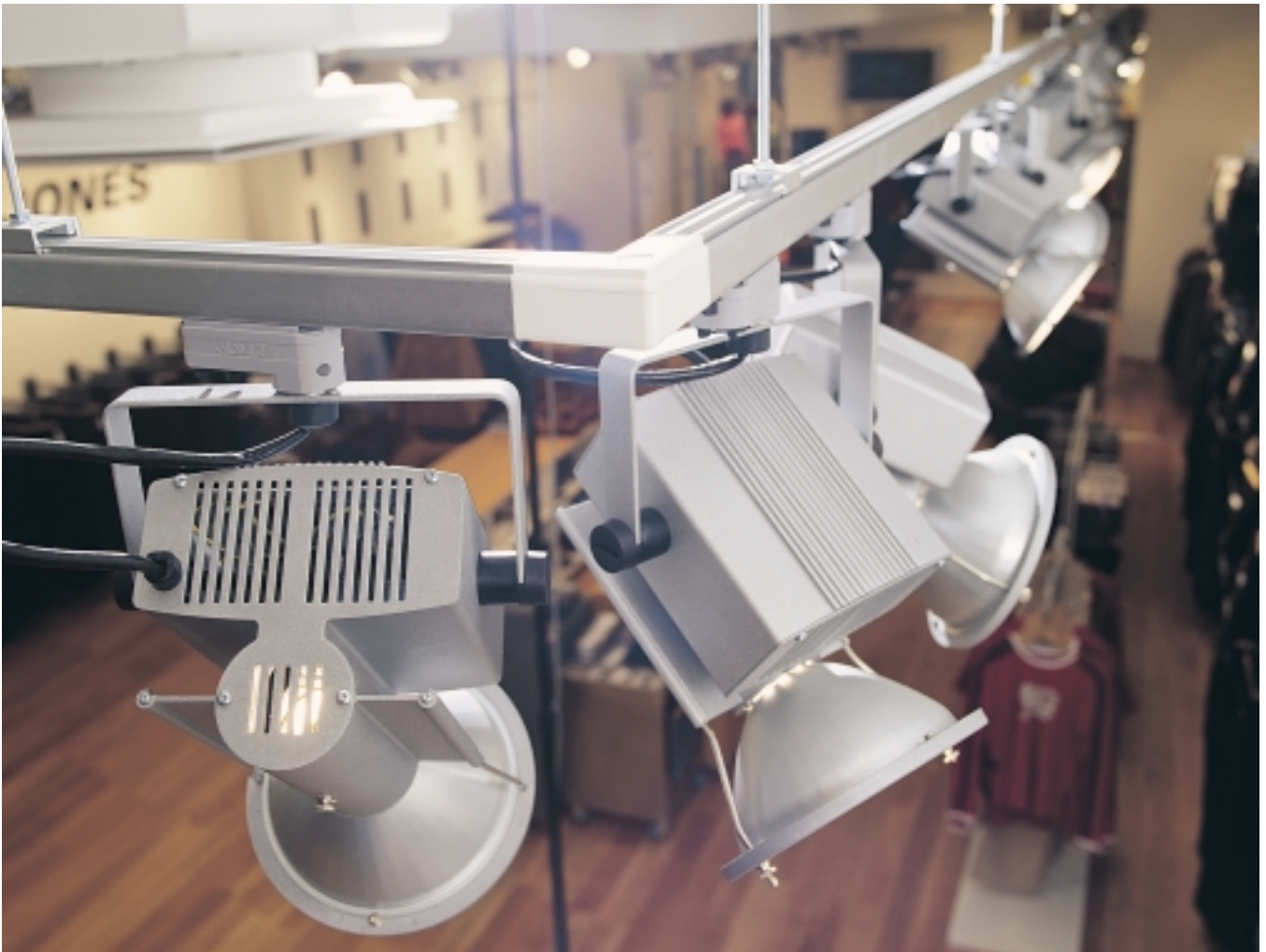
GLOBAL trac The GLOBAL trac® lighting track system allows for versatile solutions in demanding and elegant power supply applications. Light sources and power take-off points can be freely positioned exactly where required.
